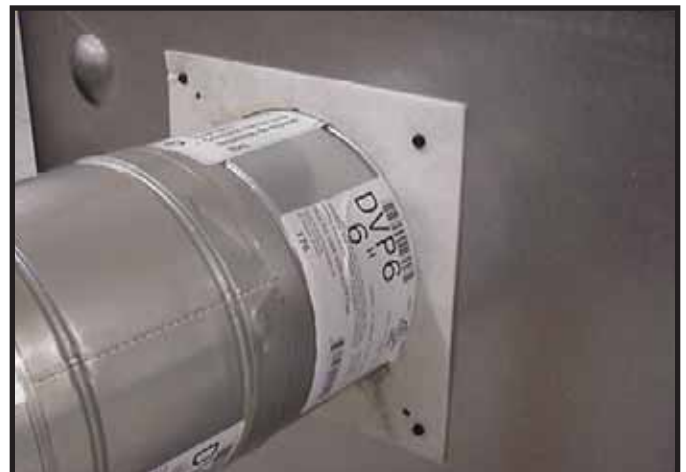
Figure 6.12 Attach the first vent section (it will snap into place). Slide the insulation gasket onto the vent section, up against the appliance and over the tabs. Use two self-tapping screws to secure gasket to outer wrap.
