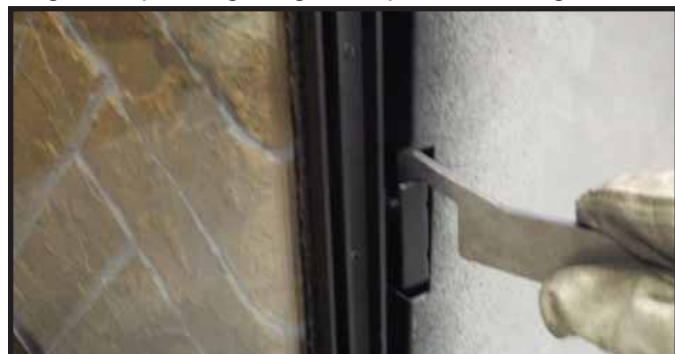
Figure 11.7. Securing Side Glass Clips
