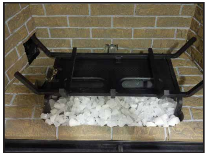
Figure 11.9. Ember Glass Area Covered with Teco-Sil
