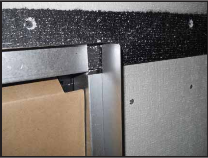
→ Figure 10.5 Finishing Template Bends
