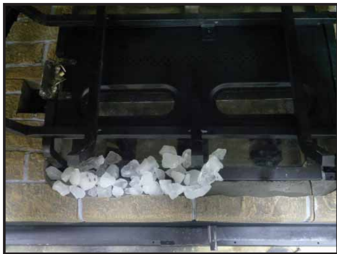
Figure 11.9. Install Teco-Sil
