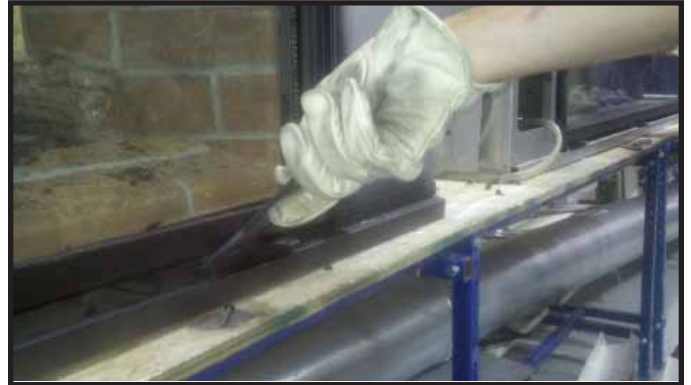
Figure 11.3. Inserting Glass Clip Tool
