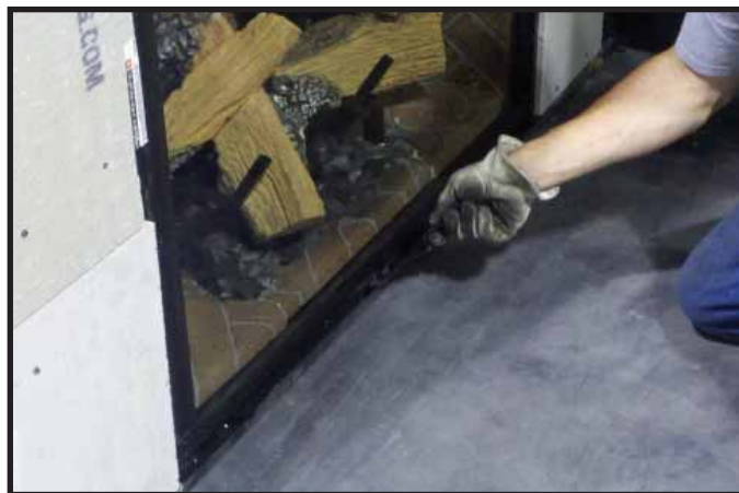
Figure 11.8. Securing Bottom Glass Clips
