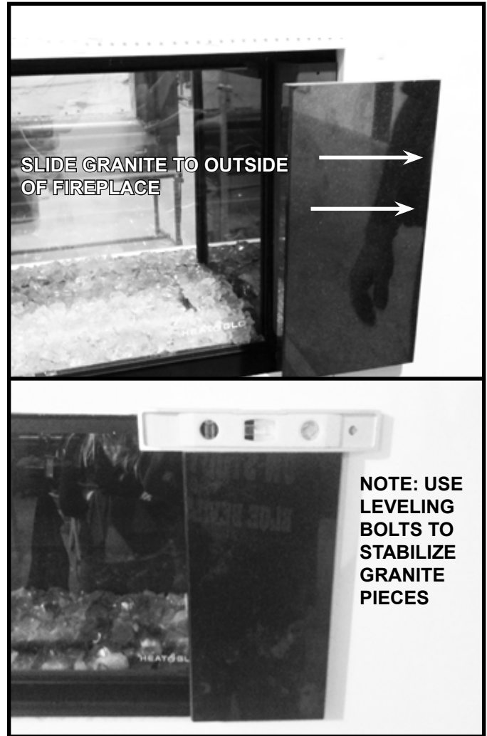
Figure 10.26. Right Side Granite Piece Installed and Leveled
