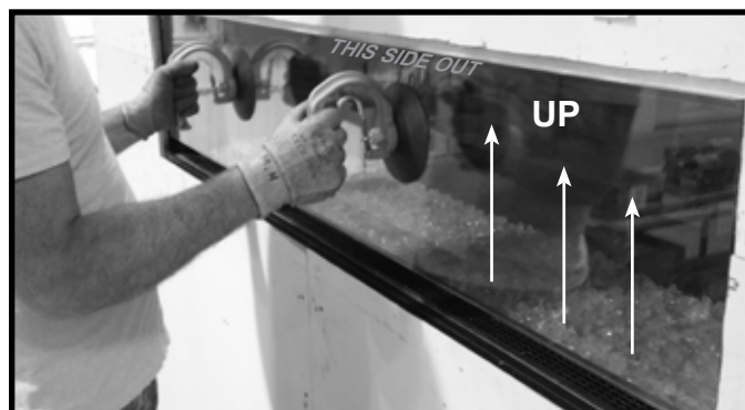
Figure 4.1 Slide Barrier Glass Up
