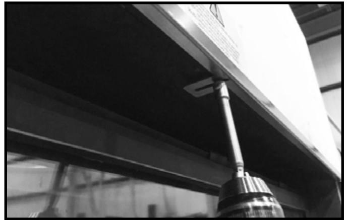
Figure 10.5. Install Trim Ring
