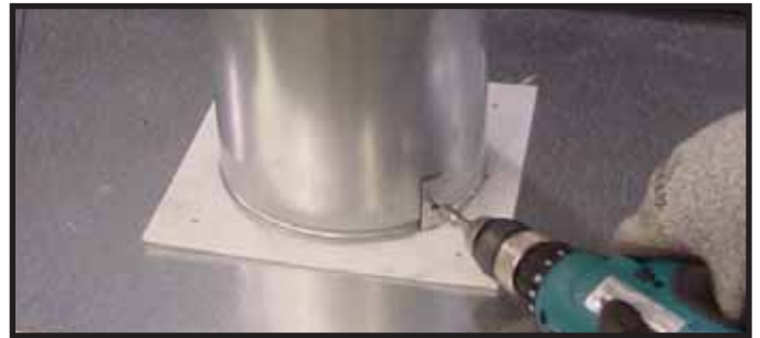
Figure 9.3 Gasket in Place
