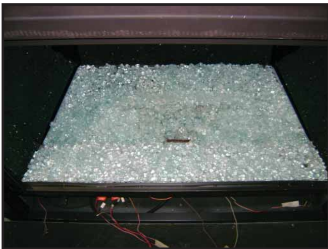
Figure 14.9 Proper Placement of Media
