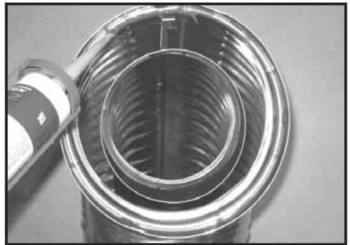
Figure 10.2 High Temperature Silicone Sealant
