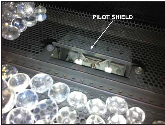
Figure 14.3. Placing Glass Rock Media on Pilot Shield
