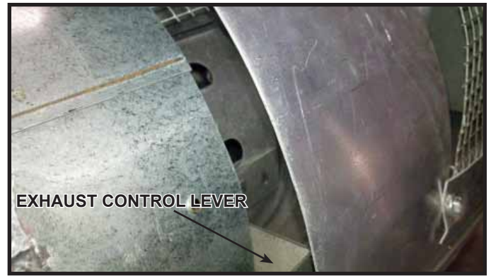
Figure 4.10 PVK-80 Control Lever Adjustment - Open
