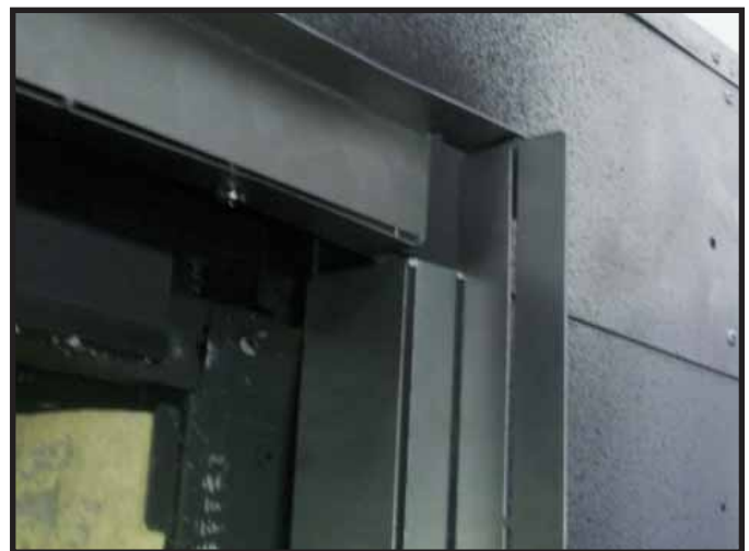
Figure 10.4 Top/Side Finishing Templates Installed
