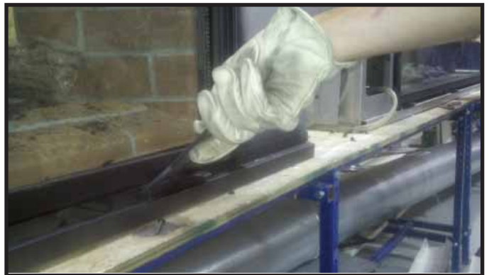
Figure 11.3 Inserting Glass Clip Tool
