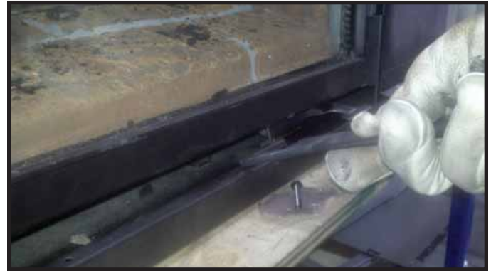
Figure 11.2 Glass Clip Tool Location
