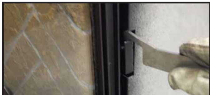
Figure 11.7. Fasten Side Glass Clips
