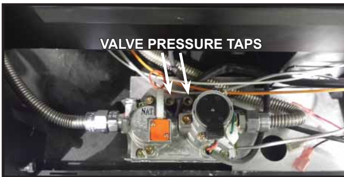
Figure 9.1. Valve Pressure Taps.
