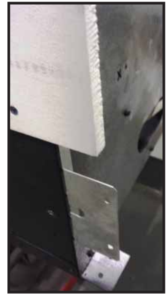
Figure 6.3 Nailing Tabs Installation Position
